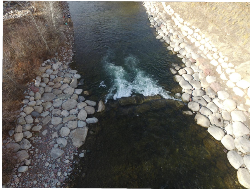
EXAMPLE OF BOULDER MATRIX PLACED TO MAXIMIZE CONTACT AND MINIMIZE GAPS BETWEEN BOULDERS
